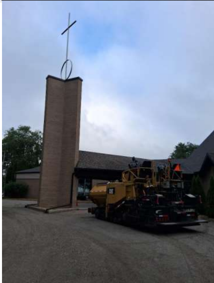
Getting ready to apply the first level of asphalt.
